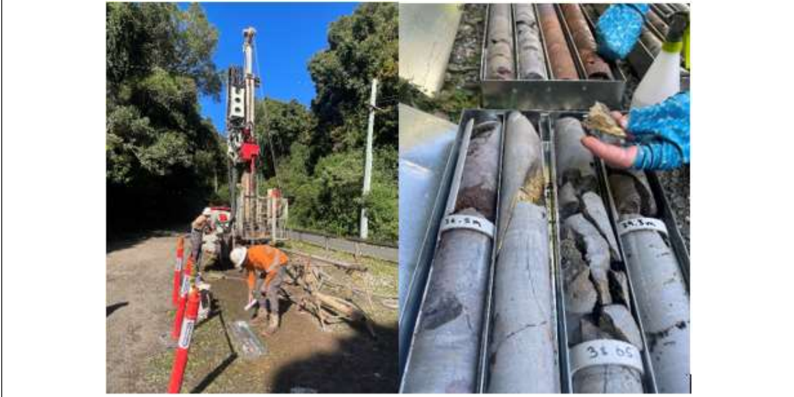
Figure 5 - Repeater Station Rd drilling rig and extracted rock core sample 2022.
